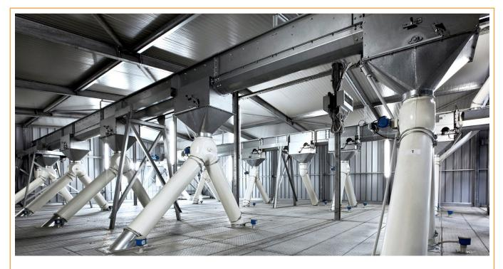
The purpose of the **PETKUS Round Bottom Chain Conveyor RF 350** is the homogenous transport of free flowing, bulky products such as grain, pulses, oilseeds and similar agricultural products.
